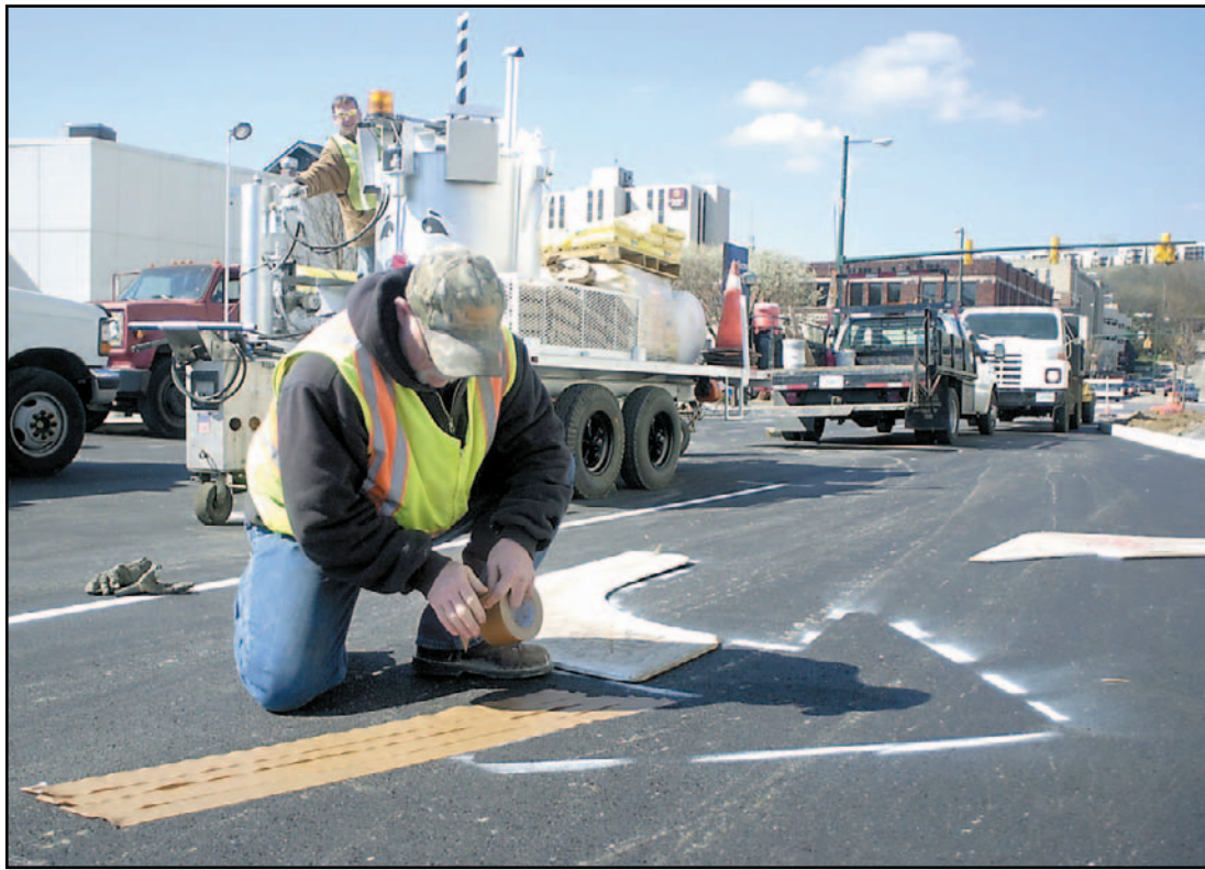
Edgar Bumgardner with Volunteer Highway Supply marks a turn arrow on Fourth Street. The street will be opened for traffic today.
